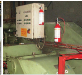
A FIRETRACE system can prevent a small fire from becoming a major event.
